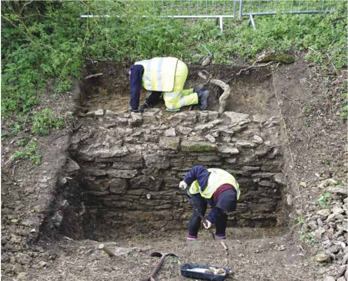
FIGURE 2 Ha-ha wall at Great Linford
