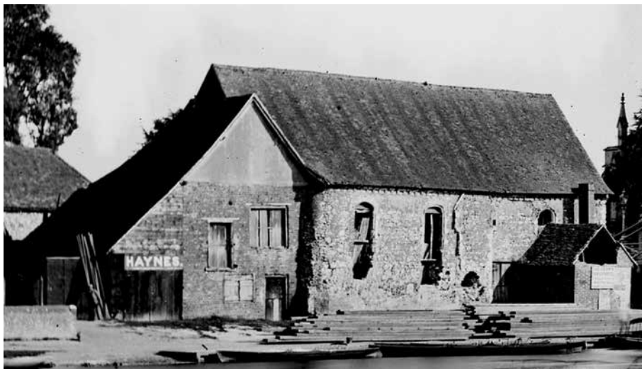
FIGURE 5 An enlargement of the Taunt photograph showing the corbel table, window design and the round-headed doorway being unblocked. By permission of Historic England Archive
