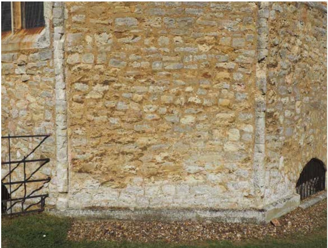
FIGURE 4 Regularly coursed masonry in ESE bay of the apse
