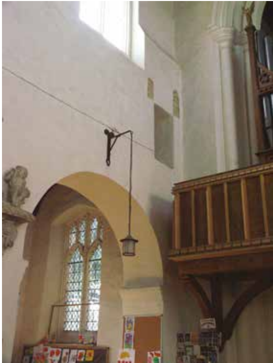
FIGURE 8 SW corner of nave showing upper doorway leading to probable former W gallery in nave
