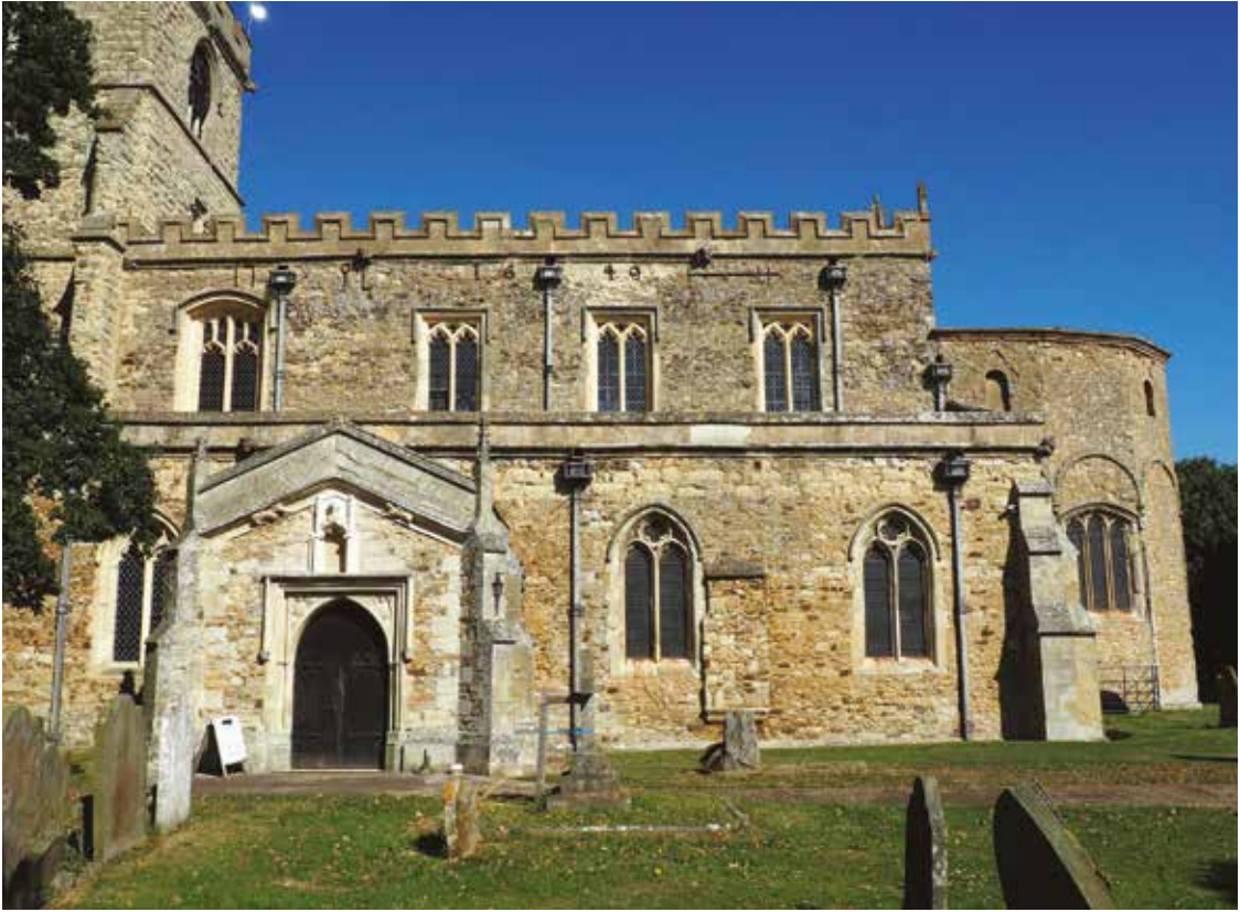
FIGURE 9 Exterior of nave and apse from S
