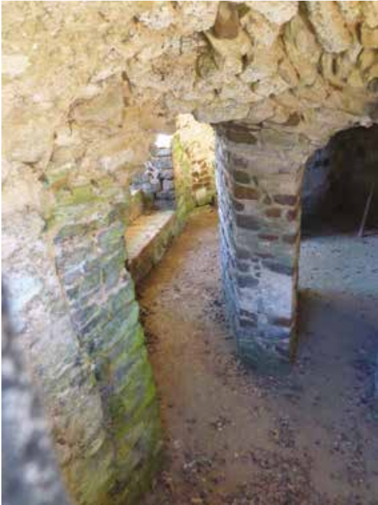
FIGURE 5 View down into crypt through E window. On left, primary jamb of niche with secondary masonry added in front to support vault; centre right, free-standing pier of added vault
