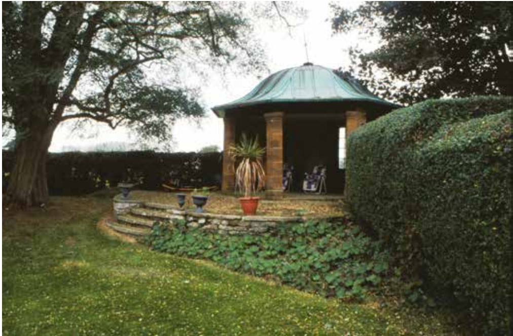
FIGURE 2 Barton Hartshorn, the summerhouse, c.1908, architect Robert Lorimer (Charles Boot/Christopher Dingwall)
