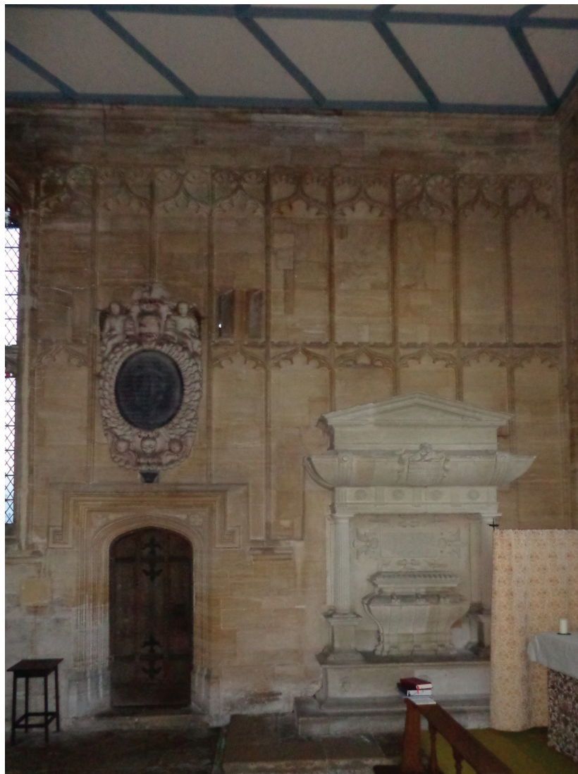
FIGURE 5 The north wall of the north chapel, showing the door to the closet and vestry block and the windows of the closet, partly blocked by the later monument above the door. ( photo: Vicki Harding )
