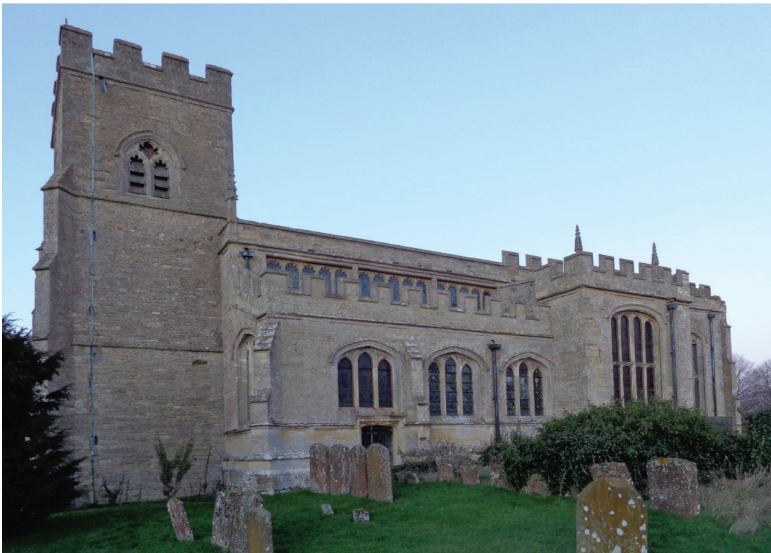
FIGURE 2 Hillesden church, south side ( photo: Vicki Harding )
