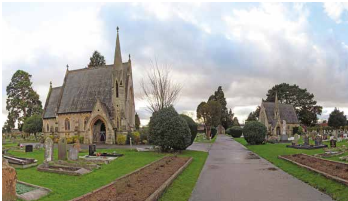
FIGURE 6 Aylesbury Cemetery: 1855, a fine layout and ensemble by architects Poulton & Woodman of Reading: the main axis, with the two chapels, leading to the mortuary, set in a good collection of C19 trees (copyright Charles Boot)
