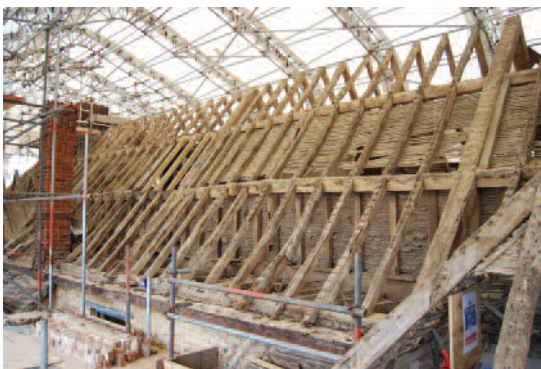
FIGURE 31 East range of the roof (looking north) after removing the tiles
