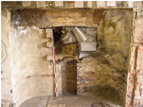
FIGURE 22 Parlour G5 fireplace showing false-jointed lining on 1790s plaster
