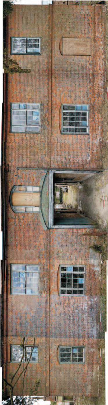
FIGURE 20 Principal elevation of the east range showing outlines of original window openings
