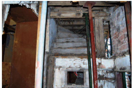
FIGURE 30 Original surviving treads for winding staircase in the southern tower
