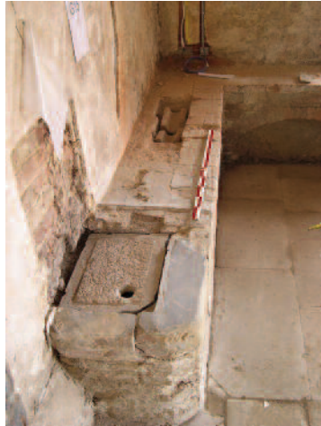
FIGURE 24 Remains of stone-lined sink and drain in the dairy
