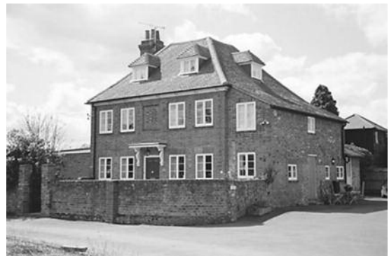
FIGURE 1 Leys Farmhouse, Thomkins Lane, Burnham, South Bucks (English Heritage Listed Building number 1124484) (photo: Carl Shillito, Images of England, record 43919)
