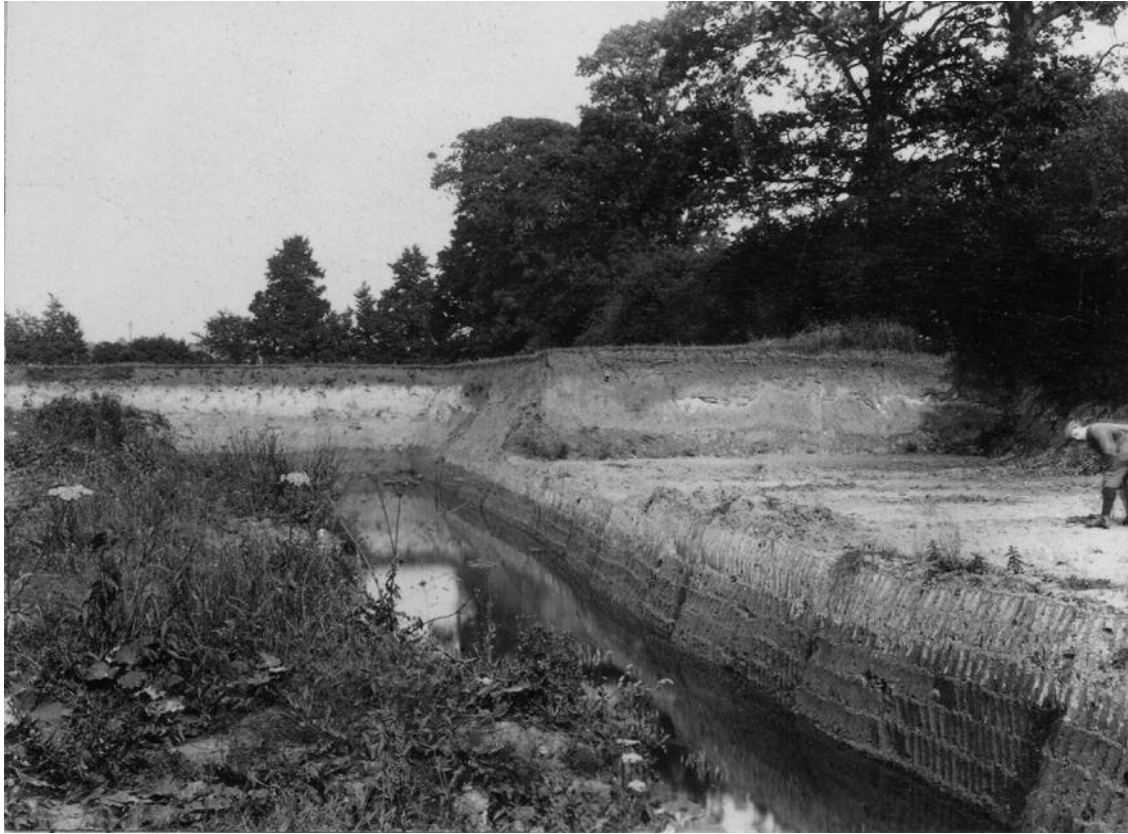
FIGURE 3 Locke's Pit, Hartwell, in 1912. The figure on the right provides some scale. The shallow alluvial deposits have been stripped and figure is standing on clay in which spade marks can be seen. Photograph reproduced courtesy the British Geological Survey, ref P252363
