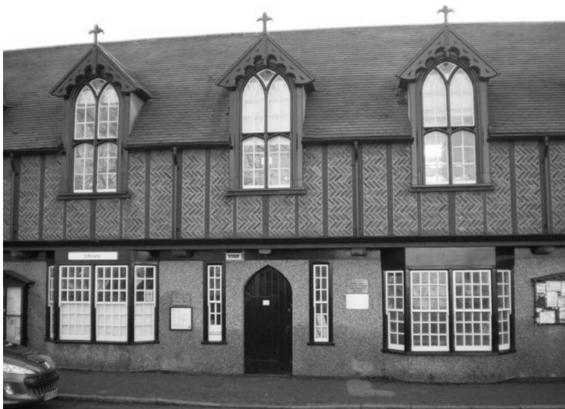
Figure 6 The former town hall at Ivinghoe, now the local library. First built in the late 16th century and originally open on the ground floor, it was modernized in the 1840s when the tall Gothic dormer windows were inserted
