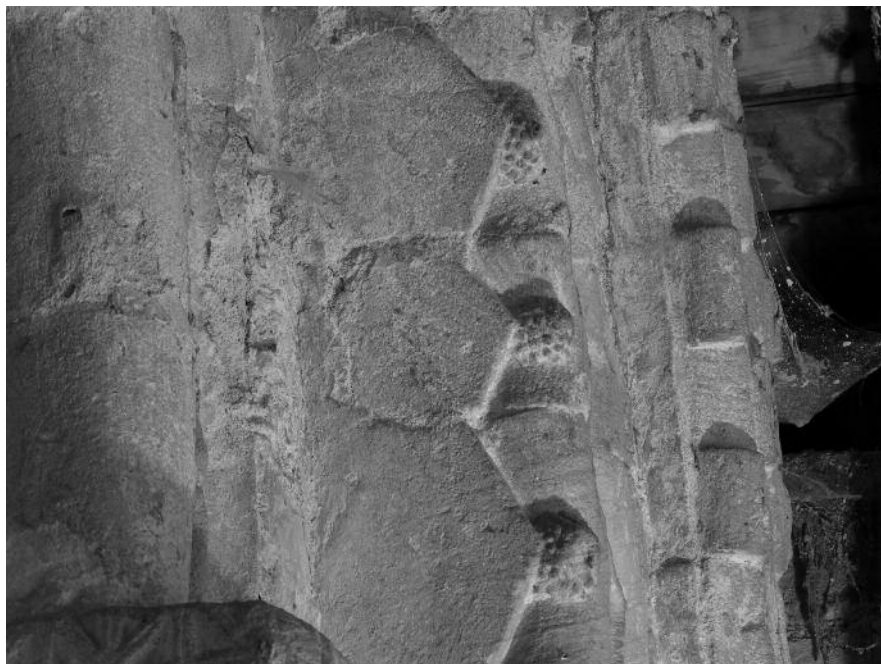
FIGURE 12 Third order: the plain soffit, the chevrons and the balls of grapes
