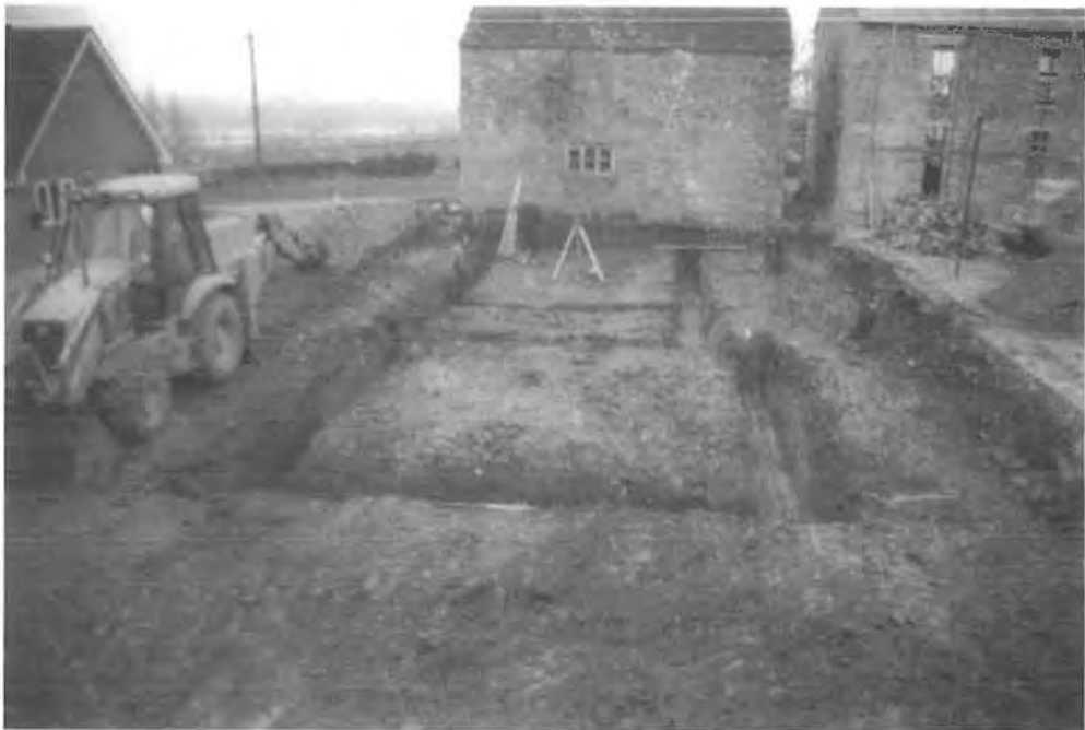
PLATE 2 Excavation area after cutting of wall footings, with granary to rear (looking south).
