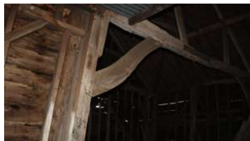
Figure 9 :Close-up of S-shaped brace in barn.
