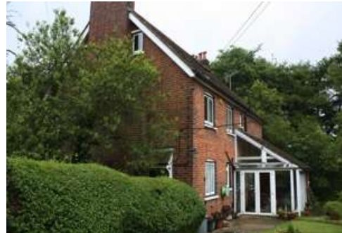
Figure 5 : Rear elevation, with the lean-to.
