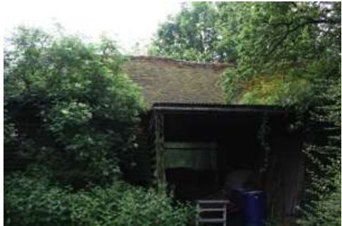
Figure 6 : The barn in overgrown farmyard.
