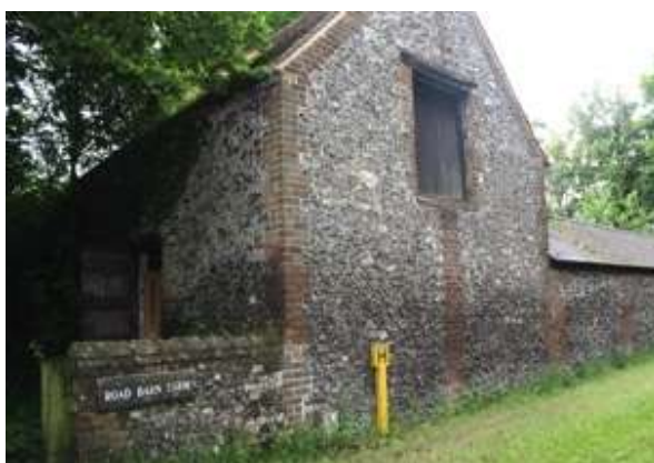
Figure 1: The roadside gable end of stable and hayloft
