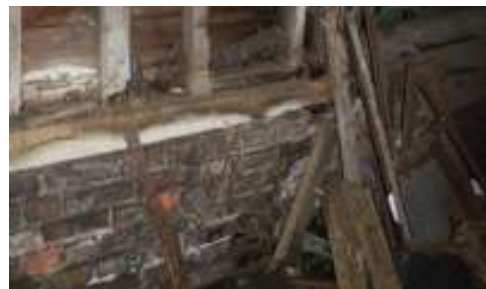
Figure 7 : The barn's high brick plinth.
