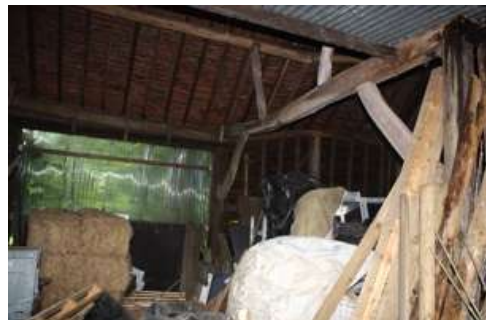
Figure 8 :Barn interior with roof truss.
