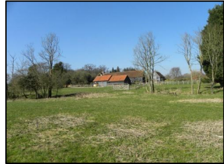
Bury Farm – the high-speed line would pass about 50 metres to the left of this picture.
