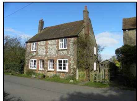
Beeway Cottage – a typical brick-and-flint labourer's cottage built with materials taken direct from the fields.
