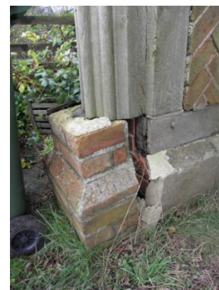
Figure 6: The brick base of one of the archway pillars.
