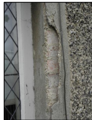
Figure 15: Exposed brickwork in the central bay.
