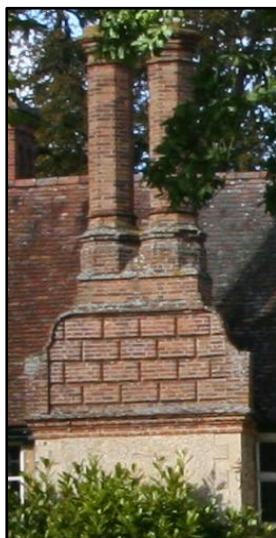
Figure 17:...and on Doddershall House.
