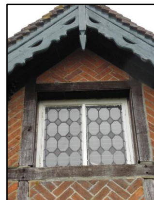
Figure 5: Octagonal leaded lights above the driveway.
