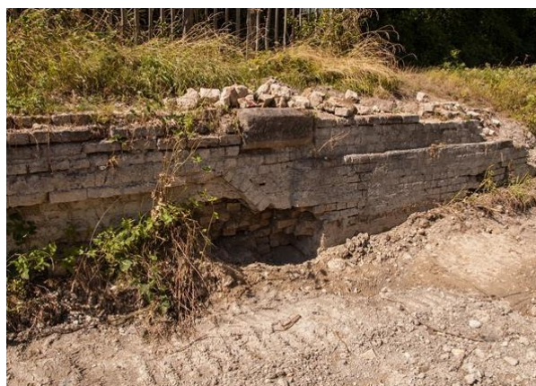
Remains of the swing-bridge abutment today.
